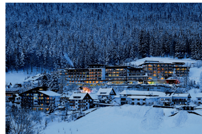
CHP for hotel "Traube Tonbach" in Baiersbronn / Germany: 2 x GC 232 N5 // Electrical power: 232 kW each // Thermal power: 358 kW each
