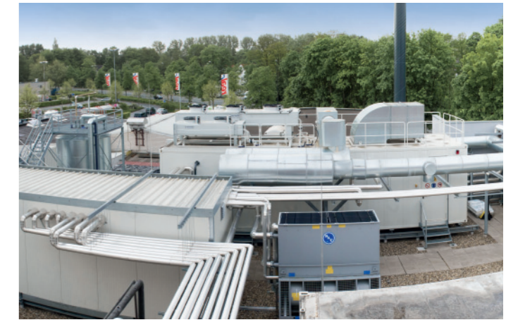
CHP for industrial bakery "Mestemacher" in Gütersloh / Germany: GR 849 N5 // Electr. power: 849 kW // Therm. power: 948 kW // Cooling cap.: 105 kW
