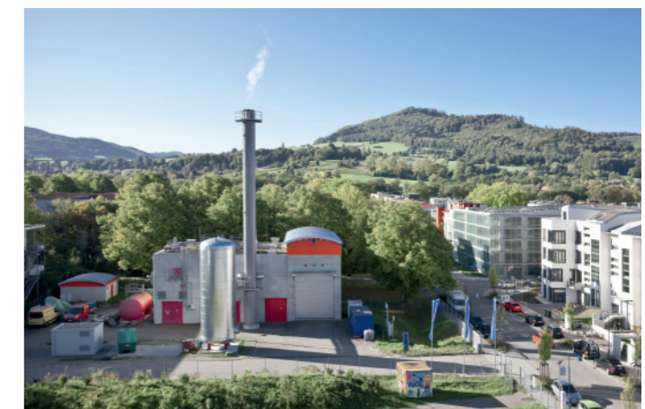
CHP for housing estate "Vauban" in Freiburg / Germany: GR 849 N5 // Electrical power: 849 kW // Thermal power: 1,300 kW
