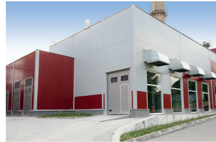
CHP for housing estate in Daugavpils / Estonia: 2 x GR 1999 N5 // Electrical power: 1,999 kW each // Thermal power: 2.2 MW each
